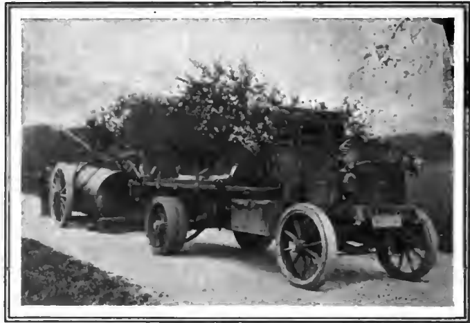
Fig. 5—Unloading the trailer of the truck
